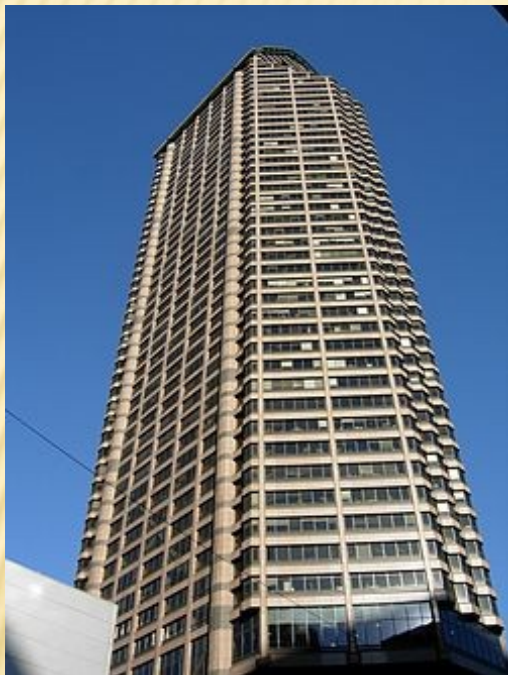
City of Seattle, WA Municipal Corporation Tower
